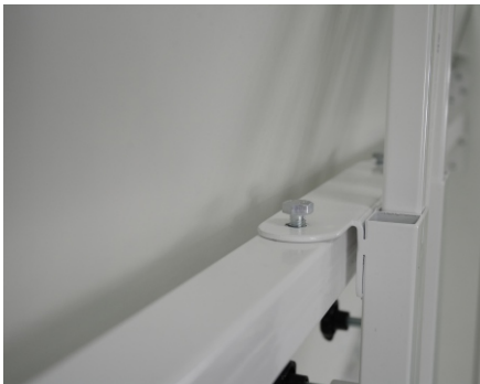
View of top crews to twist at connecting beam
